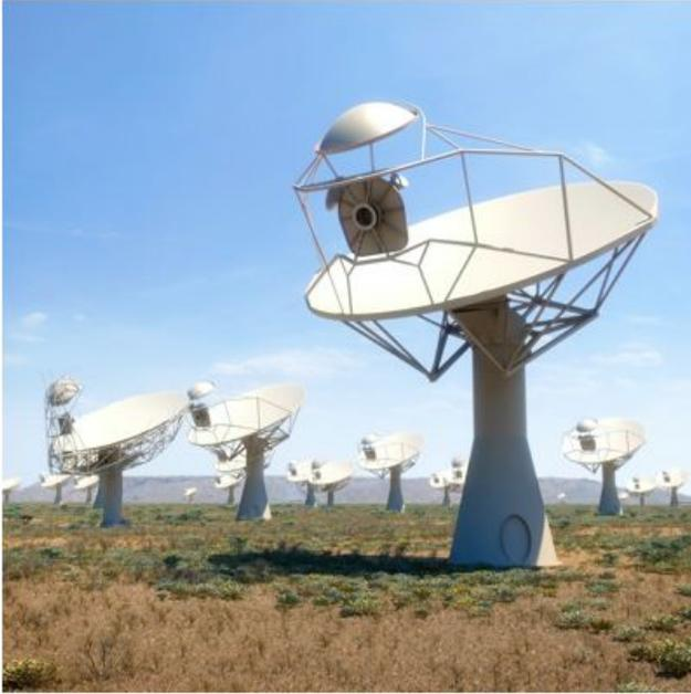
Figure 1: Artist impression of a few of the thousands of antennas that will make up the SKA. Stations of these dishes will be sited across southern Africa. They will be linked with telescopes across the continent and to Australia, making a single, globe-spanning radio telescope that is orders of magnitude more sensitive than current facilities. Image credit: SKA Organization
